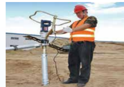
Install with drilling machine
