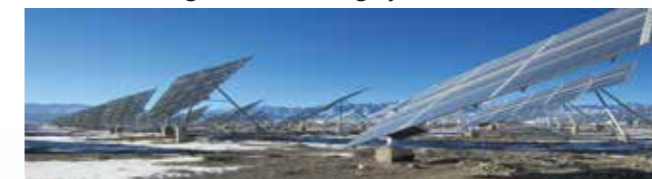
Tilted single axis tracking system
